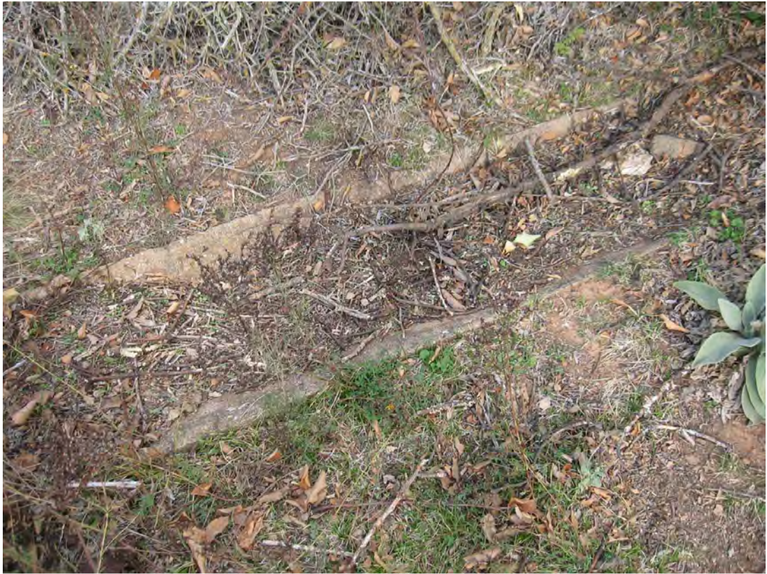
Photograph 25: Minerals processing Area – shallow concrete drain to sump structure
